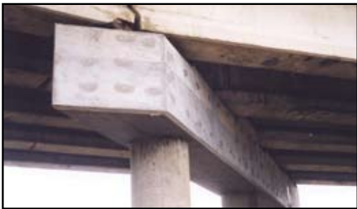
Autoroute 540/40, Quebec City, Quebec, Canada. Repair of pier cap.
