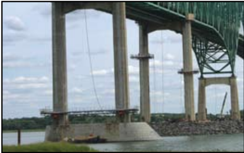
Point Lavolette Bridge, Trois Rivieres, Quebec, Canada. 10,000+ bags of SCC were used to repair patches on bridge piers that were up to 200 feet (60m) high.
